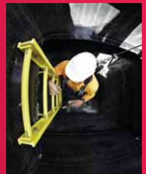
Anchoring ladder in the access chamber
