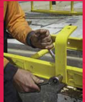
Bolting on the wall brackets
