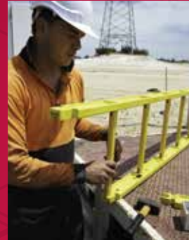
Assembling ladder to required size
