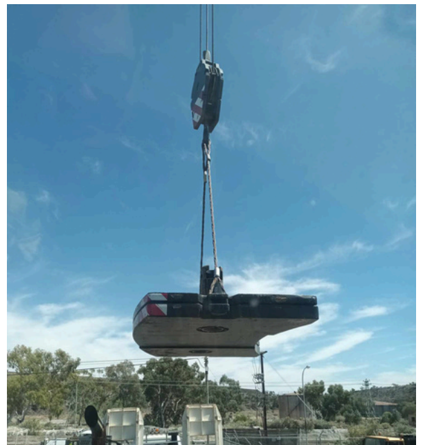
Two Ten-0 Superflex Single Slings lifting a crane counter weight.
