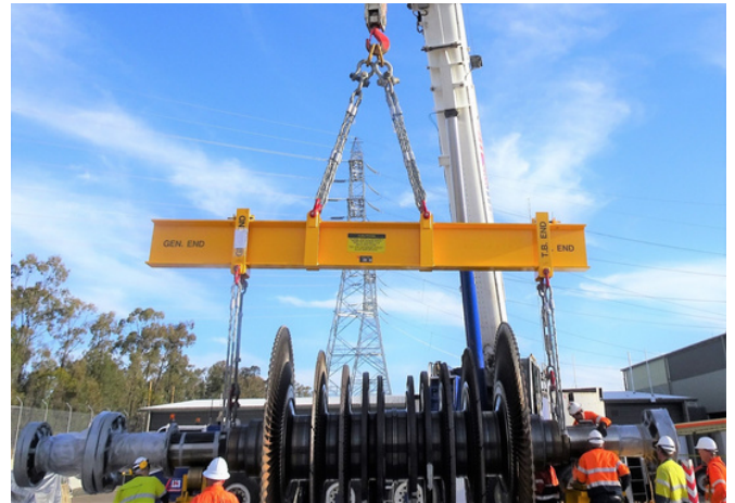
4 Double Ended stropps lifting a turbine
