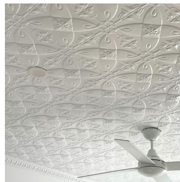
Carousel- Ceiling Feature (Painted)
