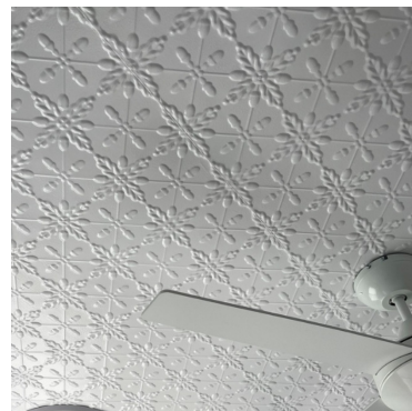
Acorn- Ceiling Feature (Painted)
