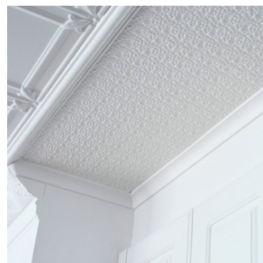
Rough Cast Small- Ceiling Infill Example
