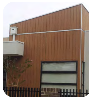
The board is continuing to lighten.
