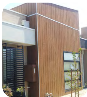
The board shows signs of lightening.
