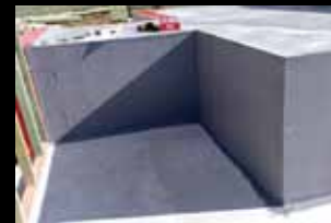
Internal wall termite and Damp-proof treatment prior to framing
