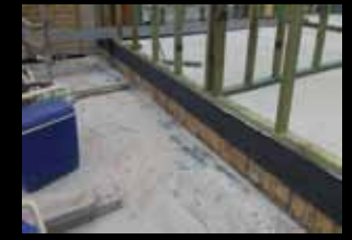
Construction Joint on step down
