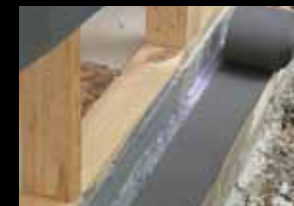
Installing PRM Cord Strip
