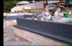
Masonry drop edge treated with coating, ant capping strip
