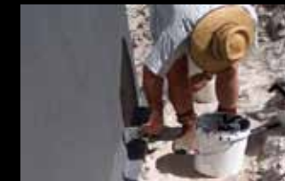
Back-Fill wall waterproofed and Termite proofed 2 in 1 application
